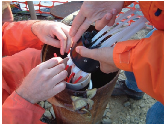
Figure 9-3 Pump Tubing Being Attached to a Wellhead
