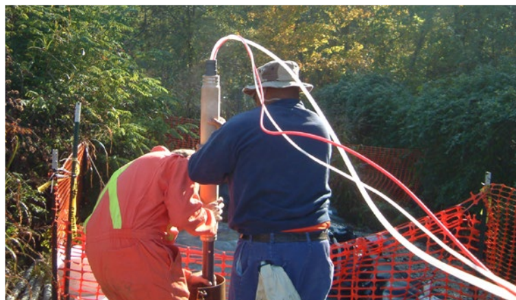
Figure 4-4 Initial Section Being Installed Down-hole
